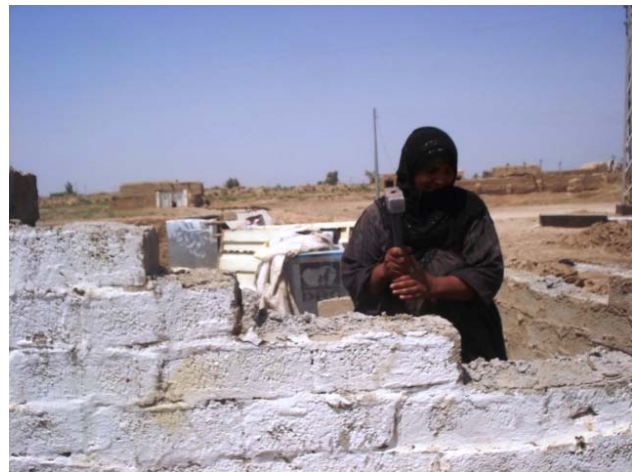
Working on House Rehabilitation in Wassit Governorate
